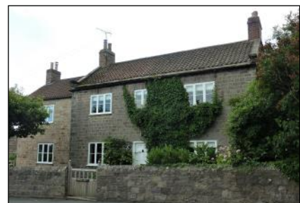
NYCVBSG 0405: Spinney Croft, Scriven. Rebuilt in gritstone about 1800 incorporating part of an earlier house with lower eaves and Magnesian limestone in the walling.
