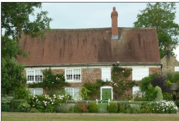
NYCVBSG 0064: Oak View, Scriven. A timber-framed house with smoke bay and 'splendid' roof, encased in brick and stone. Dendro-dated to 1516 and later. The soot on the roof timbers makes it clear that the house was built open to the roof with no upper storey, with an open fire.
