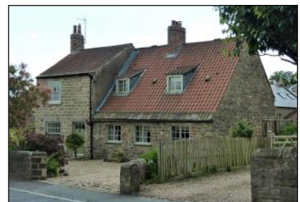
NYCVBSG 0063: Home Farm, Scriven. A timber-framed house with aisle, perhaps dating from about 1500. The report states that the present stone fireplace stands inside the frame of a timber smoke-hood, which itself was built within an earlier timber smoke-bay. At the beginning of the 17th century Home Farm underwent modernisation. The lower half of the front wall was rebuilt in stone with recessed chamfered mullioned windows, and on the back of this stone wall extending all round the north parlour a handsome pattern was painted on the plaster which includes an incomplete date of 160?. This parlour appears to have been unheated, with no fireplace.
