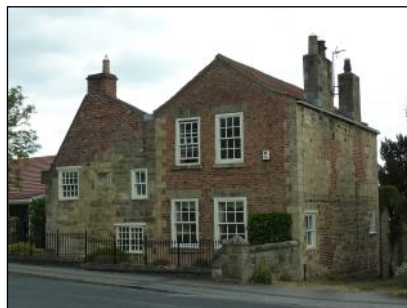
NYCVBSG 0065: Roundell's, Scriven. Consists of two separate parts: an 18th century house to the right and part of a much older house on the left. Some carved stones with part of an illegible inscription in gothic letters are built into the front wall, and a shield of arms has been set upside down in the brick wall to the right.
