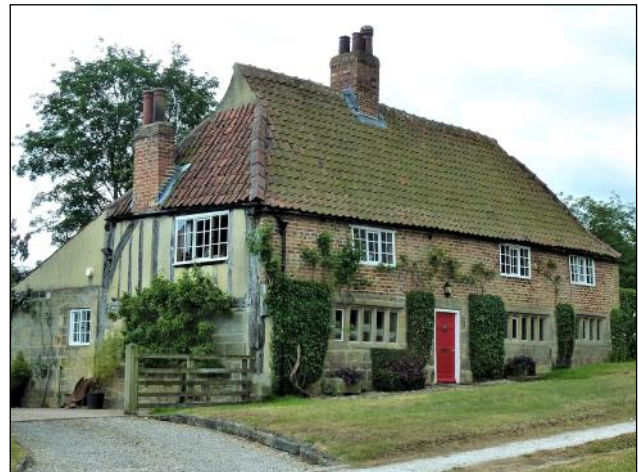
NYCVBSG 0063: Home Farm, Scriven. A timber-framed house with aisle, perhaps dating from about 1500. The report states that the present stone fireplace stands inside the frame of a timber smoke-hood, which itself was built within an earlier timber smoke-bay. At the beginning of the 17th century Home Farm underwent modernisation. The lower half of the front wall was rebuilt in stone with recessed chamfered mullioned windows, and on the back of this stone wall extending all round the north parlour a handsome pattern was painted on the plaster which includes an incomplete date of 160?. This parlour appears to have been unheated, with no fireplace.
