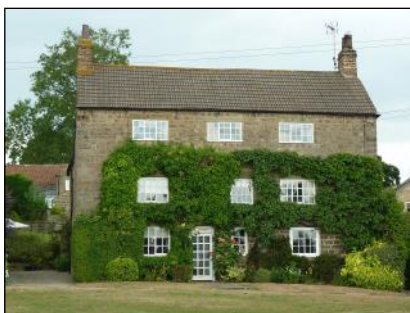
NYCVBSG 0095: Pear Tree Cottage, Scriven. Built in the 17th century with timber smokehood at each end, now removed. Kitchen in wing at rear, perhaps added to house shortly after construction. The added top floor may have been a workshop for linen weaving.
