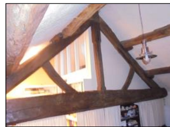
Octagonal king-post truss at Manor House, Rawtonstall
