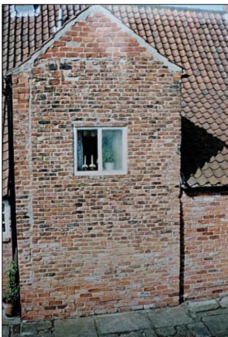
Close-up of stair turret showing long straight joint (site of post?) and altered gable, May 1994
