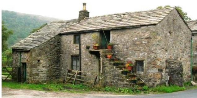
Part of Home Farm, Starbotton, before restoration as a dwelling
