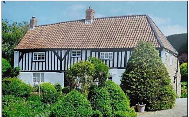
Timber framed front exterior, May 2025
