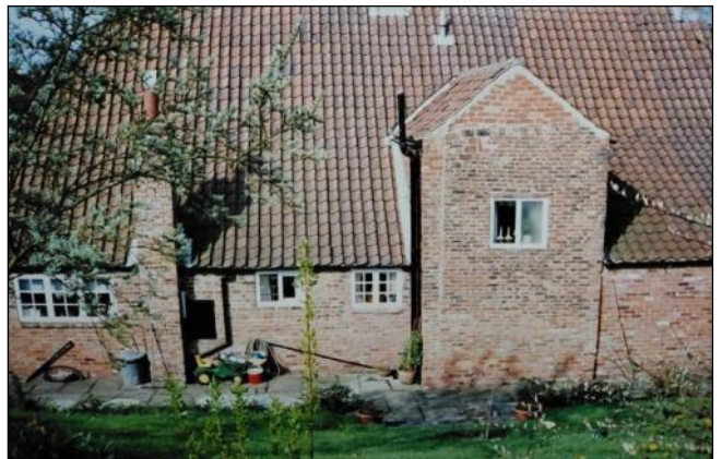
Rear elevation showing stair turret, May 1994
