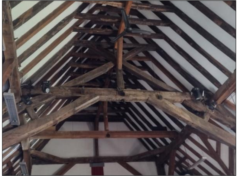
The roof at The Medieval Hall, Salisbury
