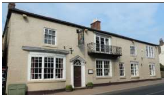
Commercial Hotel, High Street (YVBSG 0180). The early 19th century façade of this complex building hides the remnants of a timber-framed building including a beam decorated with early 16th century painting. A hollow-chamfered and broach-stopped cross-beam probably date from the late 16th century.
