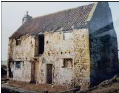
Rear elevation after demolition of rear lean-to, 1992
