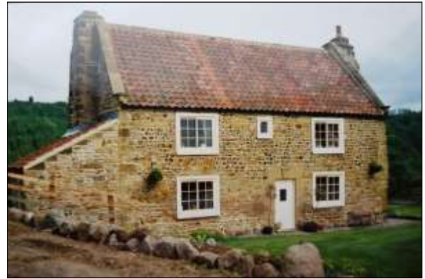
Front elevation after repair, 1994
