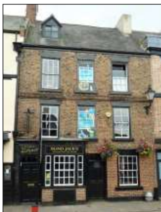
19 Market Place (YVBSG 1096). Part of a row of six shops said to be ‘newly built’ in 1611. Originally timber-framed and of two storeys, raised to three storeys with lofts in the late 17th century.
