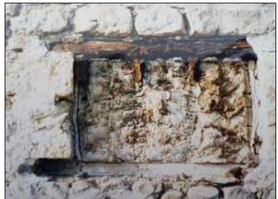
Below: Ground floor timber mullion window
