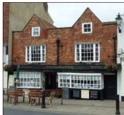
16 Market Place (YVBSG 0262). Part of a row ‘new-built’ in 1625. Timber-framed, stairs with splat balusters. Mid 18th century shop window.
