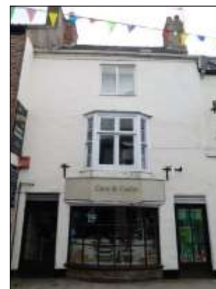
11 Castlegate (YVBSG 0163). Early example of post-timber-frame construction. Probably c1720 and designed as a shop. First floor reputed to have been used as a cockpit.
