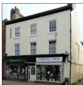
47 High Street (YVBSG 0397). This apparently late Georgian house contains the remains of a late medieval timber-framed house. Inside is a splendid ogee-arched doorway. Evidence exists of an infill of limestone chips between posts.
