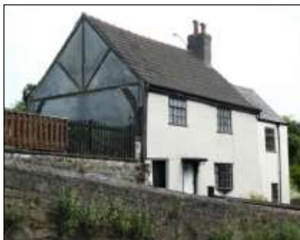
Kirkness Cottage, 35 Briggate (YVBSG 0038). A small timber-framed house, possibly mid 16th century with truncated principal rafter roof.
