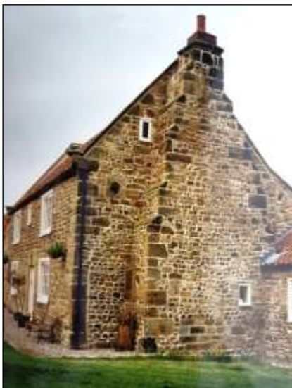
Left: South gable end, 1994
