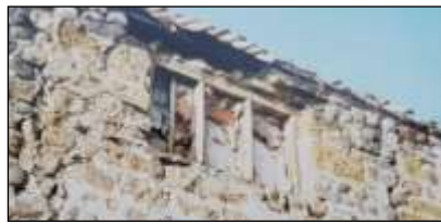
First floor timber mullion window
