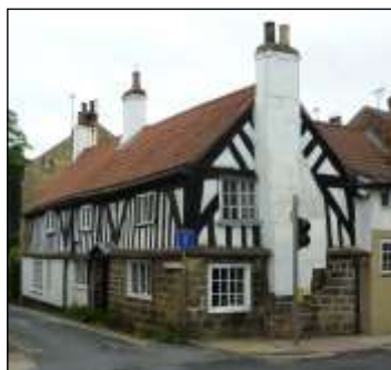
St John’s House, Church Street (YVBSG 0039). Probably 16th century with stone walling on ground floor and timber-framing above. King-post roof with V-struts. Large gritstone fireplace inserted early 17th century.
