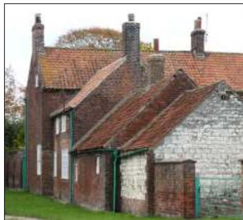
Chalk and brick buildings at Sykes Farm, Harpham, East Riding
