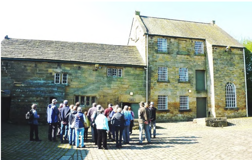
Worsbrough Mill, with seventeenth century range on the left
