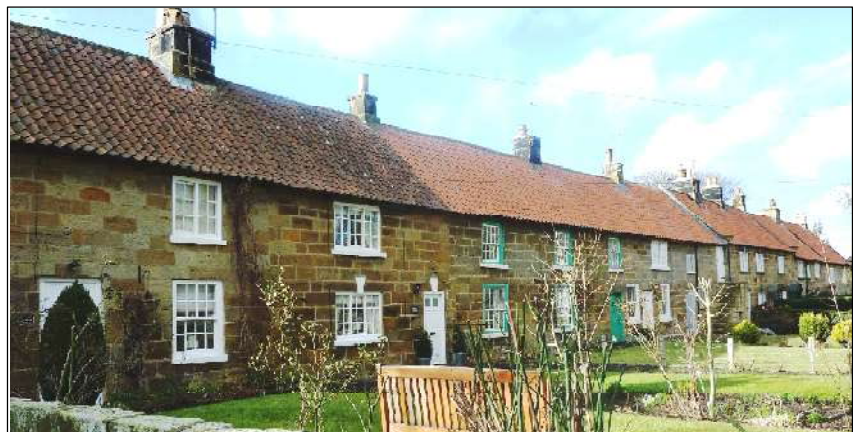
Above: Cottages in Kirkby-in-Cleveland, near Great Broughton
