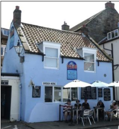
3. Sea Drift Shop (YVBSG 0926). A jointed cruck truss can be seen in the roof of this building, with the lower parts extending into a bathroom and a bedroom. This dates the building to about 1750.
