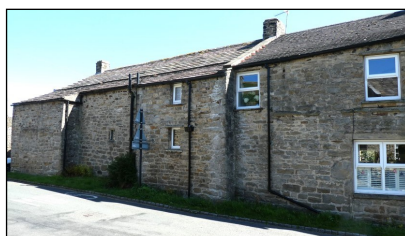
Crowtrees (YVBSG 1233). Faces south away from the road and probably dates from the latter half of the 17th century. Now two storeys but originally one-and-a-half with a steep thatched roof later replaced by stone. Inside it has two cells and single storey outshuts containing the stairs and pantry/cheese room. Divided into two cottages in the early 19th century but later reverted to one property with the original central direct entry.
