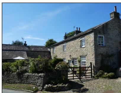
Lock Heather (YVBSG 1234). A complex of a two-cell house, cottage, barn, slaughter house, pigsties and other outbuildings, all appearing to date from c1800 and early 19th century. Partly a pub and shop at one time. Pantry lined with stone shelves for cheeses which were a major product of Swaledale throughout the 19th century.
