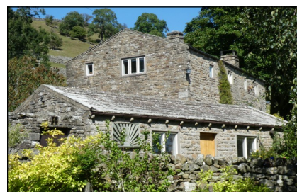
Shaw Ghyll (YVBSG 1219). Typical house plan of the area with two units (perhaps direct entry), two storeys, with an outshut containing dairy and staircase. Probably mid 18th century: external flat faced mullioned window with internal splayed jambs and chamfered mullions dateable to c1750. Extended and much altered in 1978.
