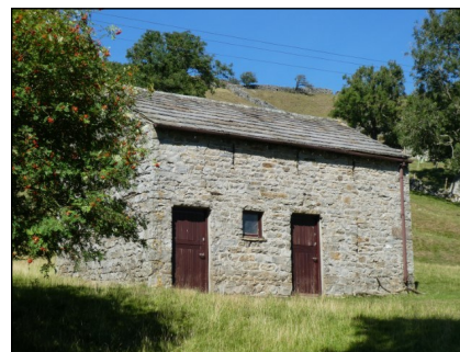
Laithe to the north of Shaw Ghyll (YVBSG 1220). The laithe is typical of the area with a division between the mewstead and the byres, with separate entrance to each. Built on a slope as a bank barn, where hay is fed into the mewstead from the higher ground level. Boskins formed from upright sandstones. Probably 18th century.
