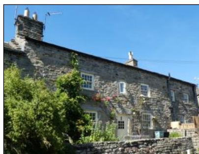
Lea House, left (YVBSG 1305) and Raisbeck House, right (YVBSG 1304). Two adjoining houses probably built around the same time with Lea House being slightly earlier, perhaps for labourers or miners rather than farmers. Almost mirror-image, sharing a central chimney stack. Raisbeck has a datestone 'SL IL 1723', maybe a later insertion. Possible re-used cruck in Lea House. Both re-fronted with 19th century watershot masonry.
