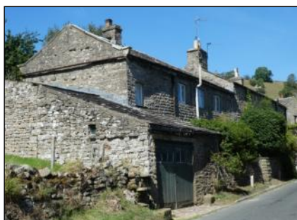
Lea House, left (YVBSG 1305) and Raisbeck House, right (YVBSG 1304). Two adjoining houses probably built around the same time with Lea House being slightly earlier, perhaps for labourers or miners rather than farmers. Almost mirror-image, sharing a central chimney stack. Raisbeck has a datestone 'SL IL 1723', maybe a later insertion. Possible re-used cruck in Lea House. Both re-fronted with 19th century watershot masonry.
