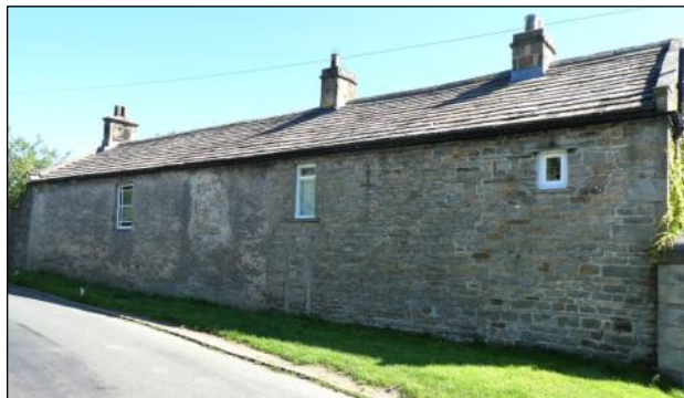
The Rookery (YVBSG 1218). Faces south away from the road towards farm buildings, now demolished. Probably originated in the 17th century, smartened up c1730-50 with new doors, panelling, kneelers, gable copings and other features. Further work in the 19th century included creation of a dairy in 1898.
