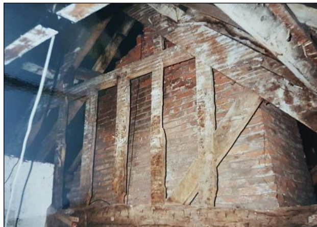
Central brick stack/smokehood with studwork in front
