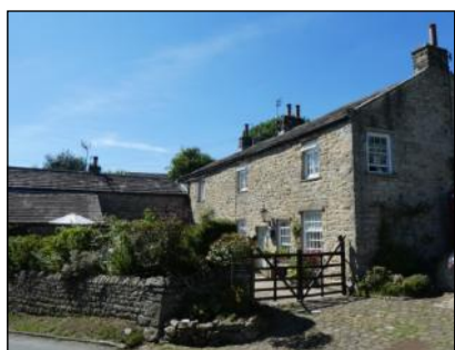
Lock Heather (YVBSG 1234). A complex of a two-cell house, cottage, barn, slaughter house, pigsties and other outbuildings, all appearing to date from c1800 and early 19th century. Partly a pub and shop at one time. Pantry lined with stone shelves for cheeses which were a major product of Swaledale throughout the 19th century.
