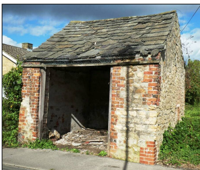
Building with roof of Harmby Slate
