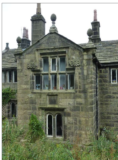
The porch at Greenwood Lee
