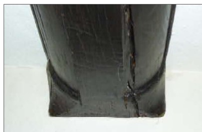
Causeway Farmhouse: ground floor beam with ovolo moulding and stops.
