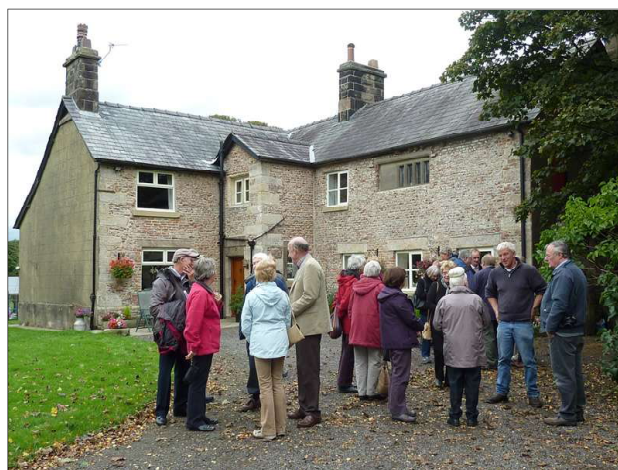
Causeway Farmhouse: a part-blocked brick mullioned window, rendered over, can be seen on the first floor.
