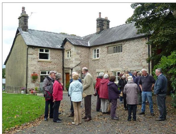
Causeway Farmhouse: a part-blocked brick mullioned window, rendered over, can be seen on the first floor.
