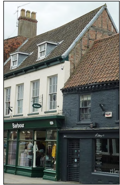
Timber-framed gable at 9 North Bar Within
