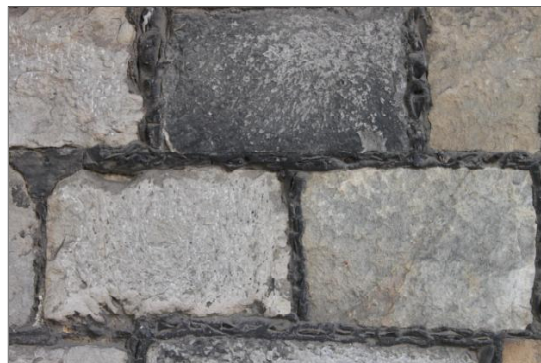
Fig 2. Nineteenth century restoration
