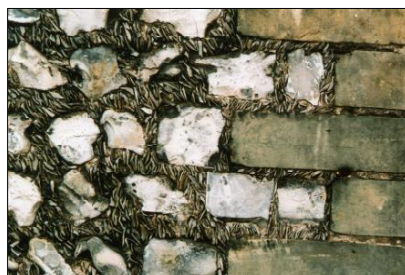
Two very different forms of masonry joint, one of flint from Sussex and the other from Dunmurry in Ireland
