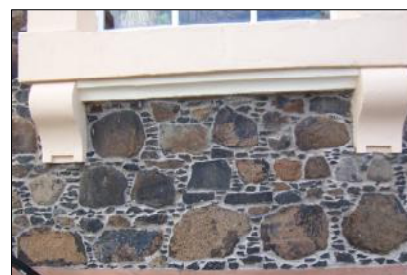
Two very different forms of masonry joint, one of flint from Sussex and the other from Dunmurry in Ireland
