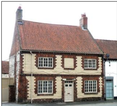
Mill Farm House, Hunmanby (YVBSG 976). A late C18 house of Georgian-style plan. Servants' room at rear accessible only by ladder from kitchen. Rounded corners allow carts to reach farm buildings behind the house.
