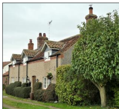
Beulah Cottage, Hunmanby (YVBSG 974). Formerly a type of longhouse with hearth-passage giving access to a cow house. Of an unusual plan in that the hearth-passage is not located behind the stack as would normally be expected. Probably C18.
