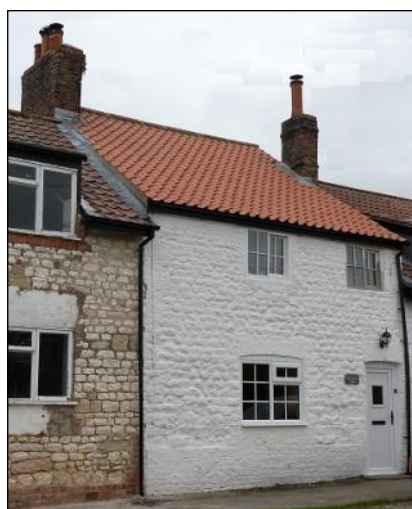
Miss Fawcett's Cottage, Wintringham (YVBSG 1001). A simple two-cell cottage of chalk and brick, probably built late C18. Yorkshire sliding sash windows on first floor.
