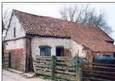
Glebe Farm, Oulton (YVBSG 1727). Cruck-framed farmhouse, a rare survival in the East Riding, dendro-dated to 1671-2. Earlier walls of less permanent material later replaced by chalk and brick. Described in full in David Cook's article in Yorkshire Buildings 35, 2007.
