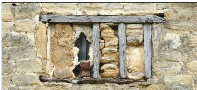
Timber mullion window seen in a barn in Hooton Pagnell
