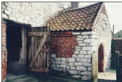
Grove Farm, Flamborough (YVBSG 1615). Chalk/brick farm buildings – barn, loose boxes/cart shed, calf house, piggery and stable – built between 1766 and 1854. Largely now demolished or converted to housing.
