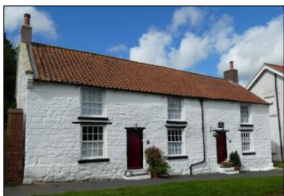
17-19 Northgate, Hunmanby (YVBSG 969). Datestone of 1694 above the door. Former three-cell through-passage plan with tall upper cruck truss above housebody. Thatch replaced by pantile c1750.
