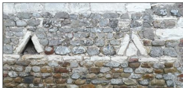
Closer view of triangular vents at Bartindale
