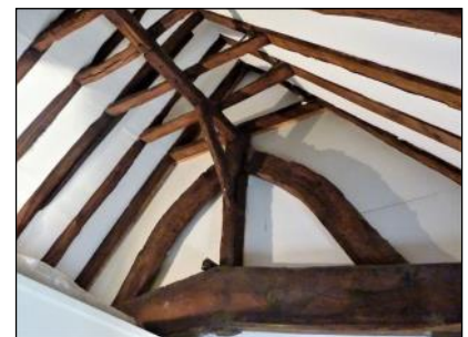
Crown post roof at 15 Flemingate, Beverley (YVBSG Report 1847)
