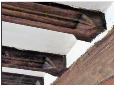
Some Yorkshire chamfer stops. Left: The Mill of the Black Monks, Barnsley; Right: Calverley Old Hall, Calverley.
