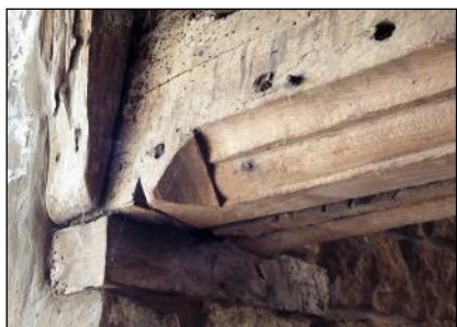
Some Yorkshire chamfer stops. Left: The Mill of the Black Monks, Barnsley; Right: Calverley Old Hall, Calverley.
