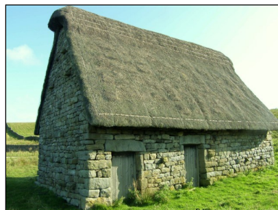
High Laithe, Grimwith (YVBSG 0278). an isolated field barn containing a raised cruck truss. 16th century but partially rebuilt 1982. Thatched with heather.
