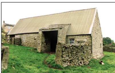
Corn barn at Drebley (YVBSG 0597). A cruck-framed barn roofed with ling thatch covered with corrugated iron. Intended for grain storage and threshing, and housing cattle at one end.
