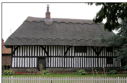
Thatched Cottage, Carlton Husthwaite (YVBSG 9 and 1885). Originally a cross-passage plan, 3½ bays with aisles at one side and one end. Perhaps 16th century.
