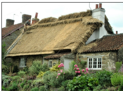
Rose Cottage, Beadlam (YVBSG 0304). Cruck-framed building, 17th century with earlier origins, acquiring a new layer of thatch from thatcher William Tegetmeier in 2005.
