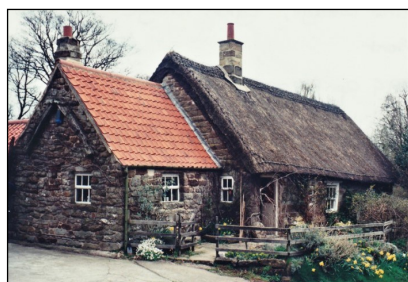
Delves Cottage, Egton (YVBSG 0309). Probably a former longhouse with byre now missing. Bressumer supported by a witch-post with St Andrew's cross and raised notched bands. Datestone on chimney 1713, presumably when smokehood removed.
