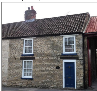
Roxby Farm Cottage (YVBSG 1766). Originally had gable facing the street. One cruck truss survives, with saddle dendro dated to 1574. Thick waney walls around the feet of crucks suggest an earlier stone plinth supporting earthen walls. Blocked fire window indicates later insertion of a firehood.
