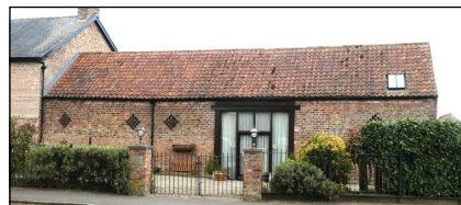
Barn at Upper Farm, Raskelf (YVBSG 1477). 17th-century brick enclosing what was deduced by one of the recorders to be a medieval three-bay timber-framed house aisled on two sides. Written up by Don McLellan in Vernacular Architecture 27 (1996).
