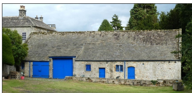
Weston Hall Barn, Weston (YVBSG 0698). A five-bay double-aisled barn. The high quality of the carpentry and the thick-section braces suggest an early date, perhaps late 15th century, with current walls dating from the 18th century.
