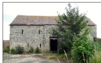
Cana Barn, Marton-le-Moor (YVBSG 1056). Built of alternate courses of sandstone and cobbles. Dating from the immediately post-enclosure period and seemingly designed for hand-threshing.
