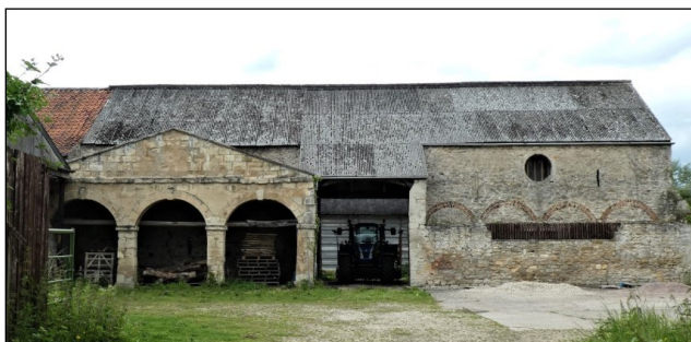
The Great Barn at Scarthingwell Home Farm, Saxton (YVBSG 1067). A twelve-bay barn built of Magnesian Limestone, containing thirteen roof trusses. Part of a model home farm probably built around 1770.
