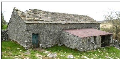
Battersby Barn, Selside (YVBSG 1815). A Ribblesdale laithe with a shippon and a hoghouse. The hoghouse is relatively recent and was built as a shippon, converted for use by sheep in the 20th century. In the barn is a remarkable collection of graffiti which includes drawings of ships.
