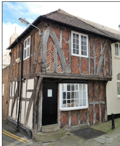
Old Dog and Duck, 45 Quay Street (YVBSG 1650). A fragment of what was once a larger building, perhaps forming a single building with 47 Quay Street. The moulded jettied bressummer is decorated with brattishing, similar to York examples.
