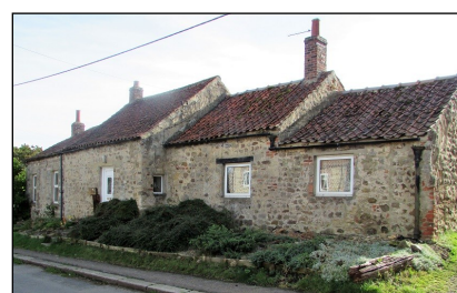
Little Owl Cottage (YVBSG 1580). The curving lines of the rear stone wall suggest the influence of at least two cruck trusses.
