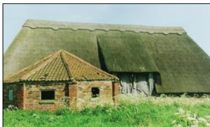
Tithe Barn, Easington (YVBSG 1544). Apparently a late 18th century structure built from two earlier timber frames which have two distinct orders of carpenters' marks, one to either side of the threshing floor. Horse engine house added after 1855.
