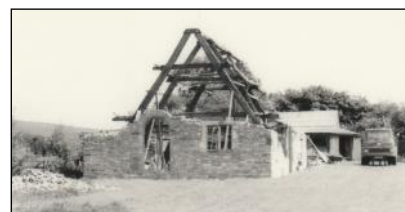
Old Manor House, Harome (YVBSG 0316). Three full cruck trusses. Dendro-dated to 1530-57. Relocated in 1971 to Ryedale Folk Museum where it is open to the public.
