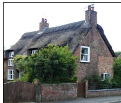
Thatched Cottage, Tockwith (YVBSG 1011). Thought to have been built originally as a 'Vale of York' type of timber-framed house with one aisle and three bays of more or less equal length.
