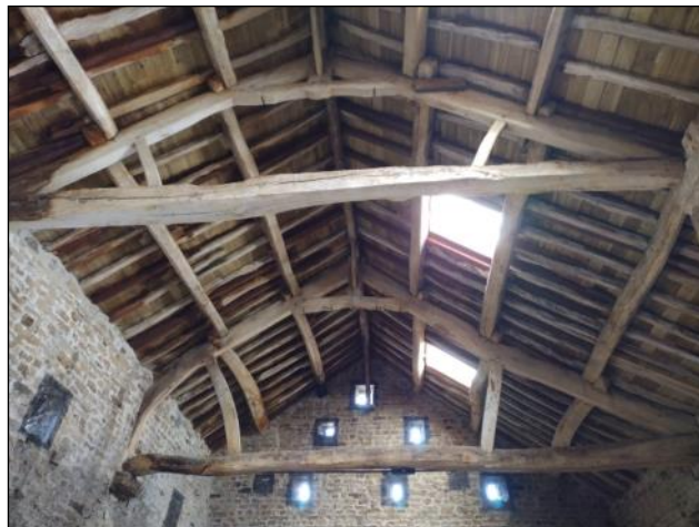
Two of the barn's five roof trusses
