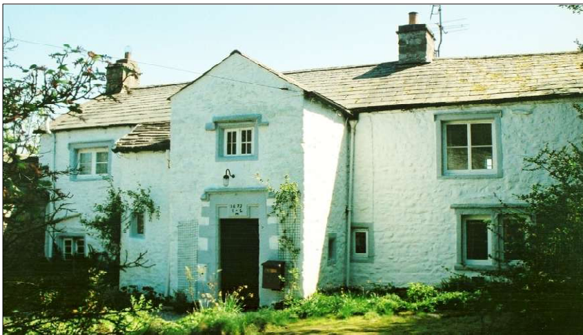
Battle Hill Farmhouse, Austwick, dated 1673 on battlemented lintel, with curved staircase turret in an unusual position at the front!
