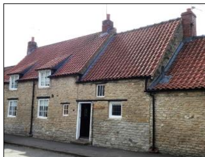
Cruck Cottage, formerly Dixons Cottage (YVBSG 1773). Had at least three pairs of crucks (dendro date of 1512), probably with earthen walls on a high stone plinth and with a thatched roof. Main housebody floored over in late C17 and fine hooded fireplace assembly inserted. In C18 or C19, part of byre was converted to a kitchen which remained open to the roof, while the rest of the byre remained in agricultural use for some time.
