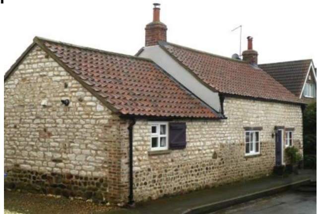
3 Pump Lane, Bempton. Chalk rubble cottage built on cobble foundations. The listed building description mentions a single roof truss with a tie beam which is a reused cruck blade, the two principal rafters possibly also being cruck blades.
