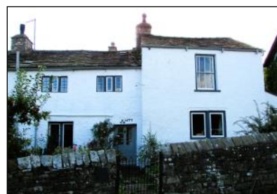
Toft's House (YVBSG 367). There are two porches which have been added onto Toft's; one is much larger and more finely built than the other. It has an arched door, with a small arched window above it. There have been numerous phases of development at the property.
