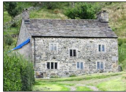
Coombe House (YVBSG 368). When Coombe was visited in 1977 it was in a state of disrepair. The stone chimney had fallen in and the remains of a lathe and plaster firehood were visible on the upper floor. The building is currently being renovated.
