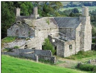
High Hall (YVBSG 543). High Hall is unusual in terms of having large stacks with round caps. It is currently in a state of considerable disrepair. However, a large plaque with Latin inscription, apparently dated 1665, is still in situ.
