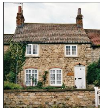
Next Door (YVBSG 1575). This single cell cobble and boulder cottage is adapted to the very narrow site between two other buildings. Internally, two cambered hardwood tiebeams may originate from an earlier building.
