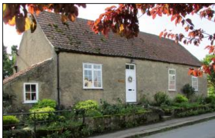
Springfield (YVBSG 189). A single storey three cell house with rendered rubble stone walls and three pairs of crucks internally, with saddle apexes (Type C). This may have had a hearth-passage plan form but has been much altered over the years.
