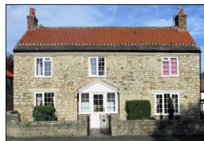
Greenways (YVBSG 1602). Changes in the front wall and quoining suggest this house was originally another single storey structure. As at Braeside, there was originally a cross passage running from front to rear doors.
