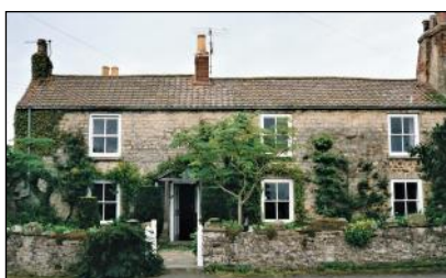
Old Village Farm (YVBSG 1574) was most likely a low cobble-built three unit farmhouse. In 1772, the date over the front door, the house was raised and significant alterations made.
