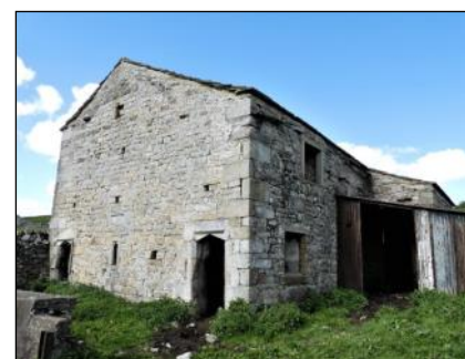
Sedber Barn, Grassington (YVBSG 1230). A field barn close to Linton Falls, with the elevation facing the river having ornamental door lintels, jambs and ventilator slits. Datestone of 'HW 1682'.
