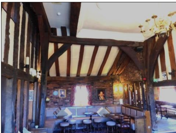
The Old Hall, Heckmondwike: the open housebody, view towards rear aisle, with inserted plaster ceiling.
