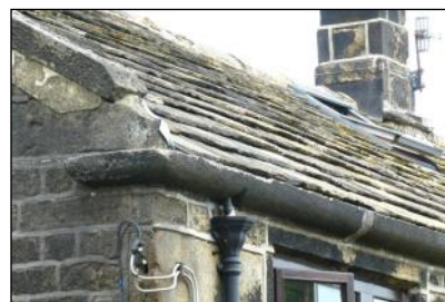
Stone guttering at 7 and 8 Higher Langfield Cottages
