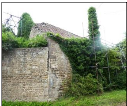
Beacon Farm, Flamborough (YVBSG 1616). A brick and chalk barn probably dating from c1770, later modified to become part of a foldyard complex. Evidence of a lower steeper roofline. Decorative ventilator slits.
