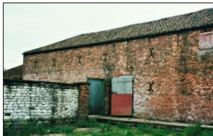
Beacon Farm, Flamborough (YVBSG 1616). A brick and chalk barn probably dating from c1770, later modified to become part of a foldyard complex. Evidence of a lower steeper roofline. Decorative ventilator slits.
