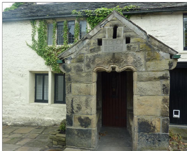
Porch at Manor House, Wilsden
