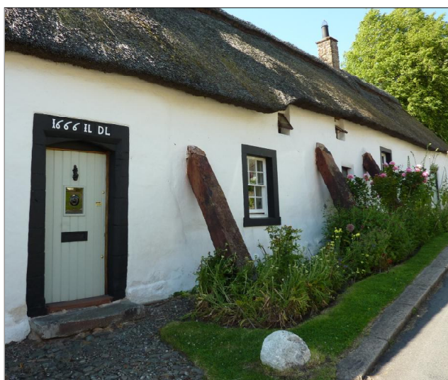
Meadowbank, West Curthwaite – a clay dabbin
