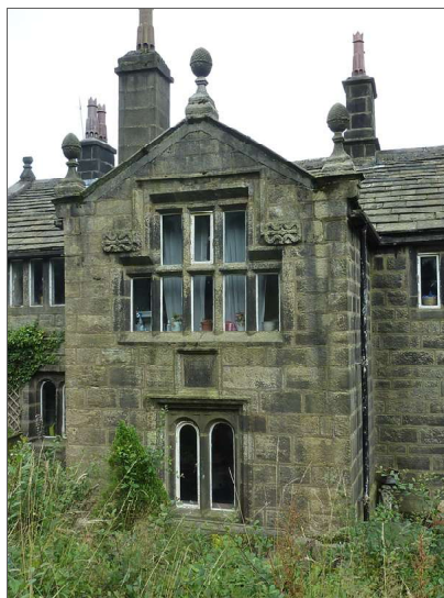
The porch at Greenwood Lee
