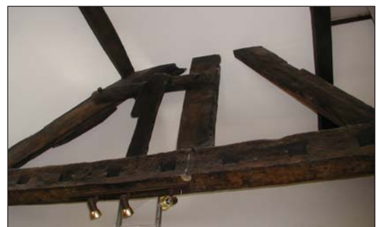
Roof timbers at Field Head Farm
