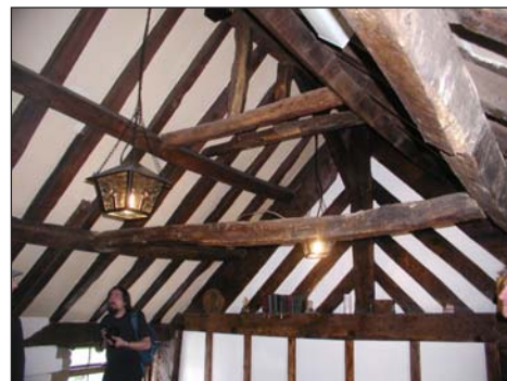
The timber structure in the roof at Brampton Hall
