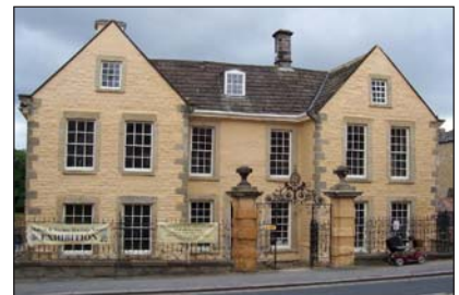
Front view of York House
